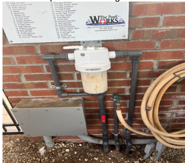
Pool air valve repaired.
